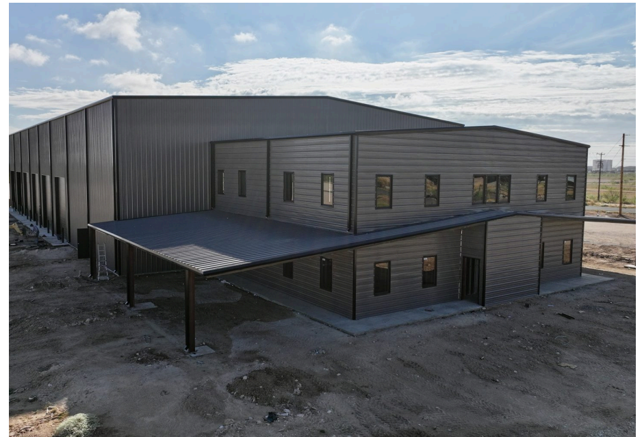
Two-story office with wraparound covered parking
