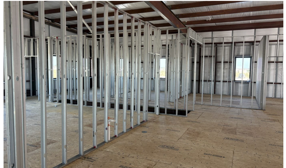
Break area and restroom plumbing
