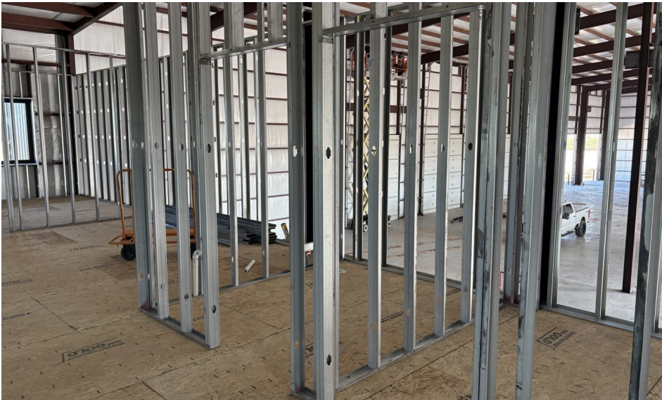
Office looking into the shop
